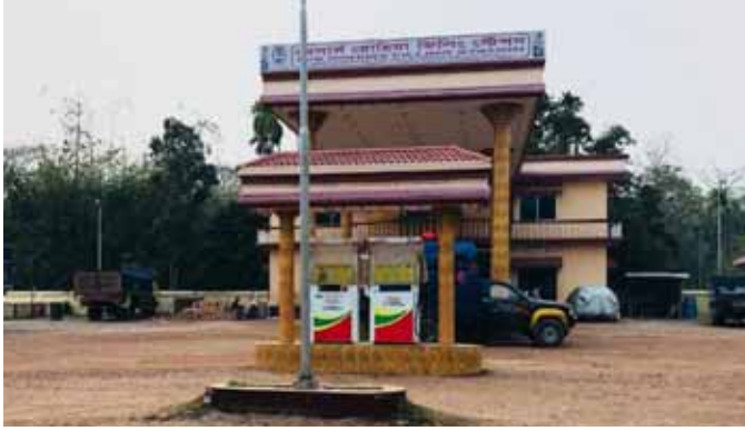
Project Name: Rohima Filling Station
